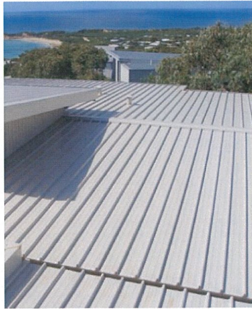
Powdercoated steel roof sheeting, cappings, guttering, downpipes, flashings .
