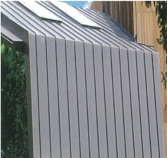
Vertical Metal cladding to Library Canopy.
