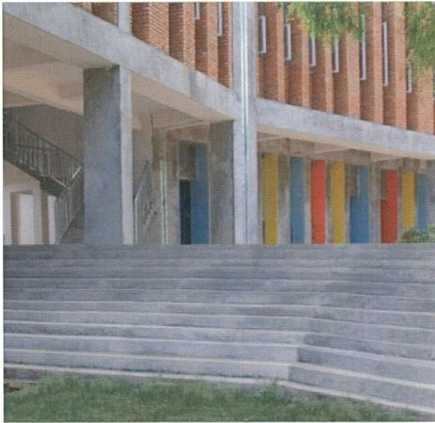
Exposed Off-form concrete structural elements including columns, slabs, soffits and balustrades.
